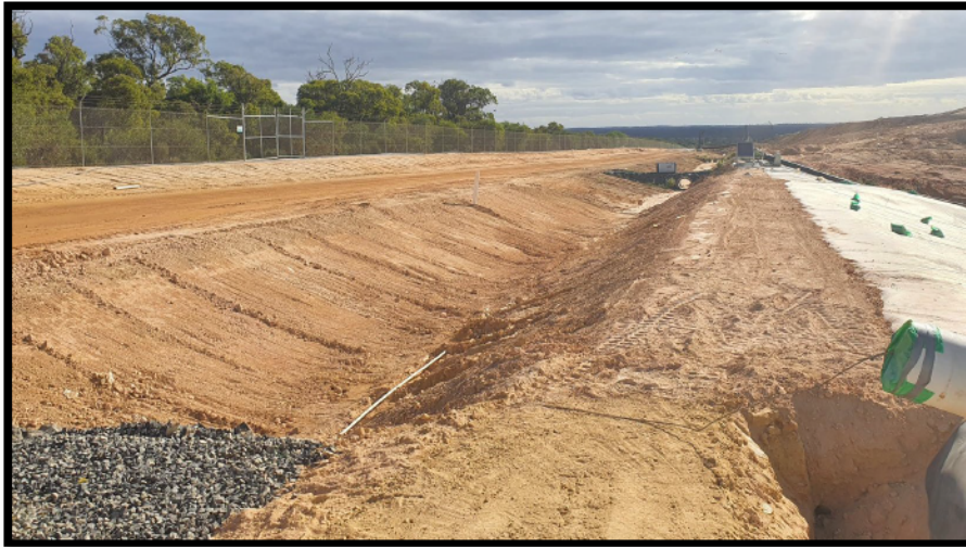
Plate 1. Cyclone fencing on southern property boundary and upgraded stormwater infrastructure.
